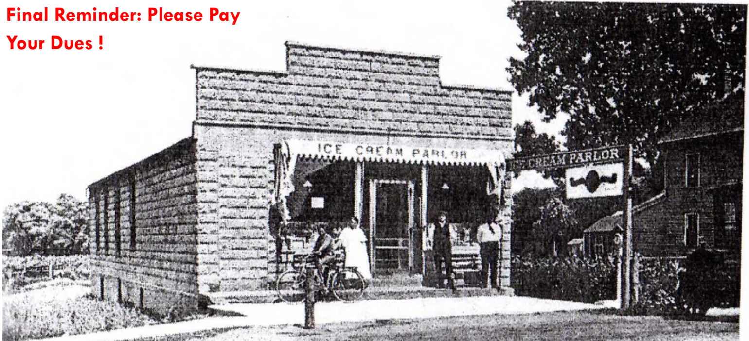
JENSEN's ICE CREAM PARLOR on Milwaukee Ave. was built by the Utpadels, using cement blocks for which they were famous.
